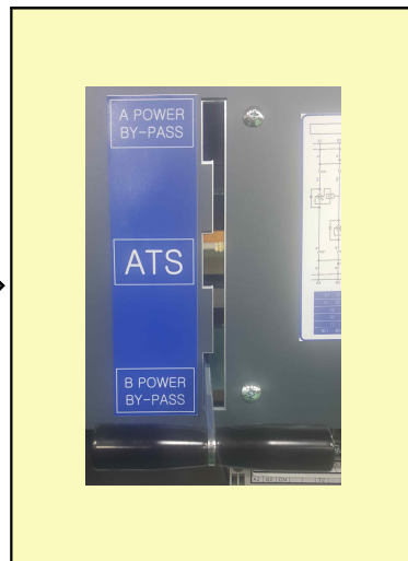
- Move the operating lever to the "B" power By-pass position.
