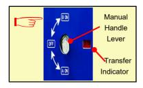
③ Transfer the switch by using and turning Manual handle lever to B-ON(clockwise)
