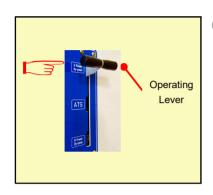
② Select "Operating Lever" so that Main ATS and By-pass Switch are parallel.
