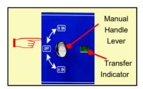
① By-pass Switch should be positioned at OFF position.
